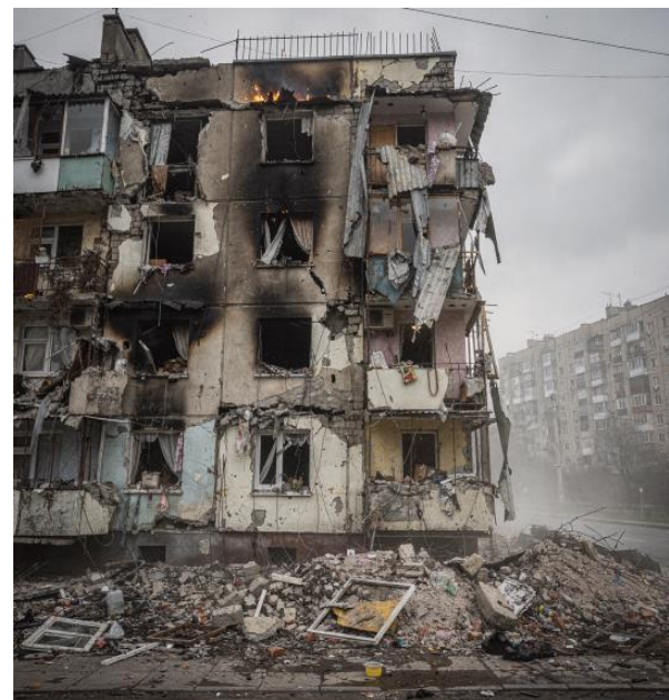
Fig. 2. Façade destruction in residential building, Kyiv (example of moderate to severe damage classification)
